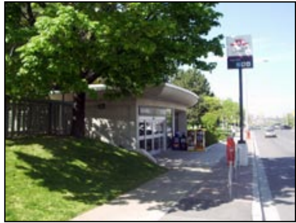
Existing Don Mills Subway Station
