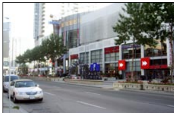
Midrise building scales tower to street
