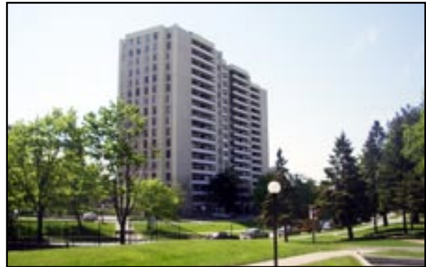
View of existing building
