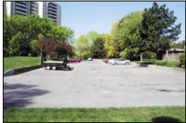
Existing grade related parking at Parkway Forest
