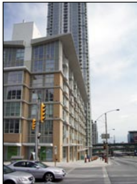
Midrise building scales tower to street
