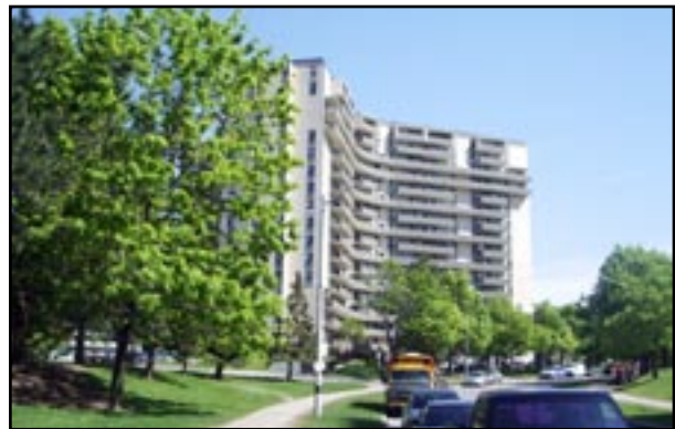
View of existing building
