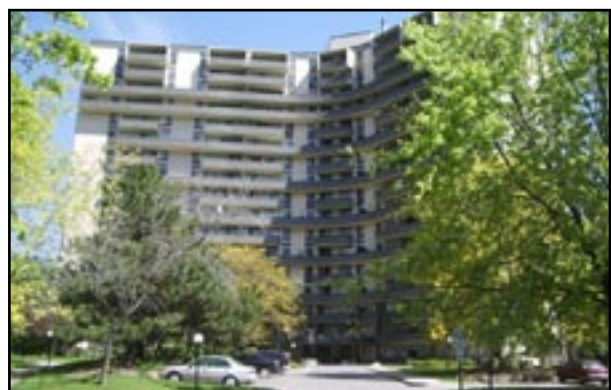
View of existing building
