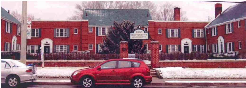
1365 Bayview Avenue: Kelvingrove Apartments
