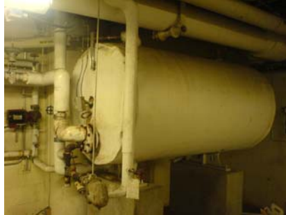
Mechanical Room DHW storage tank beside condensate return lines and tank for pre-heating.
