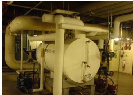
Tank and pumps in Mechanical Room #101
