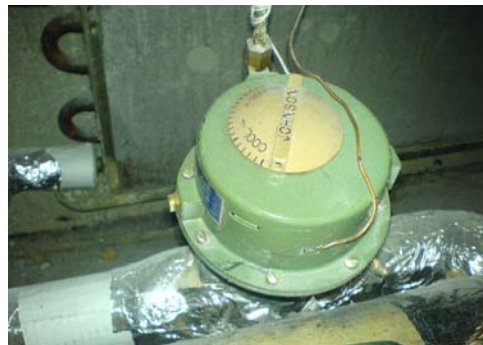
Close-up of induction unit control valve and manual control dial
