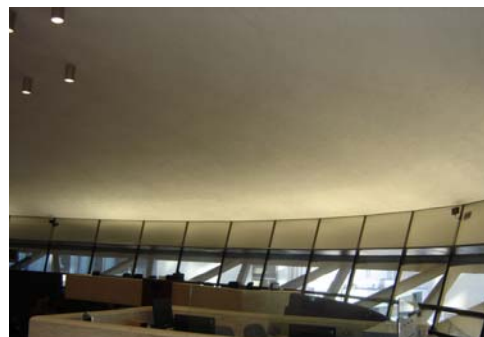
Council chamber perimeter lighting
