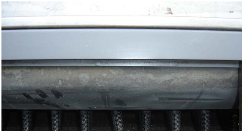
Top view of exposed induction unit nozzles
