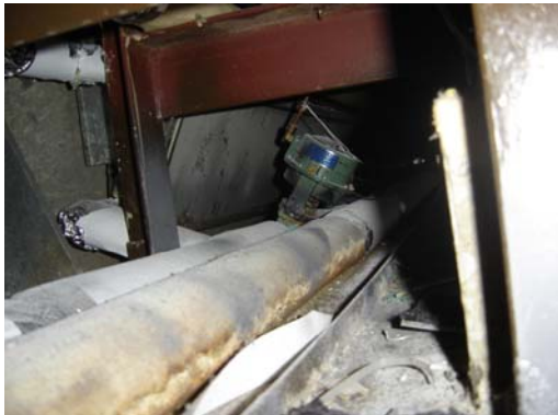
Typical induction unit pneumatic control valve, 6 – 8 per floor
