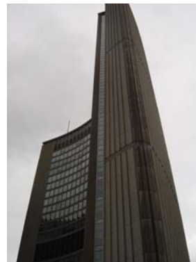
East tower "rib" showing vertical stairwell windows to be fitted with BIPV
