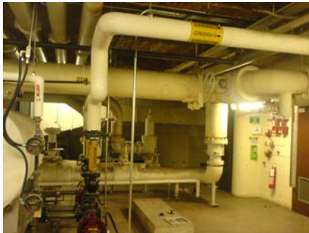
Main condensate line.
