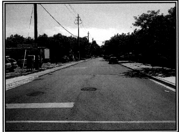
THORA AVENUE SOUTHBOUND AT DANFORTH AVENUE
