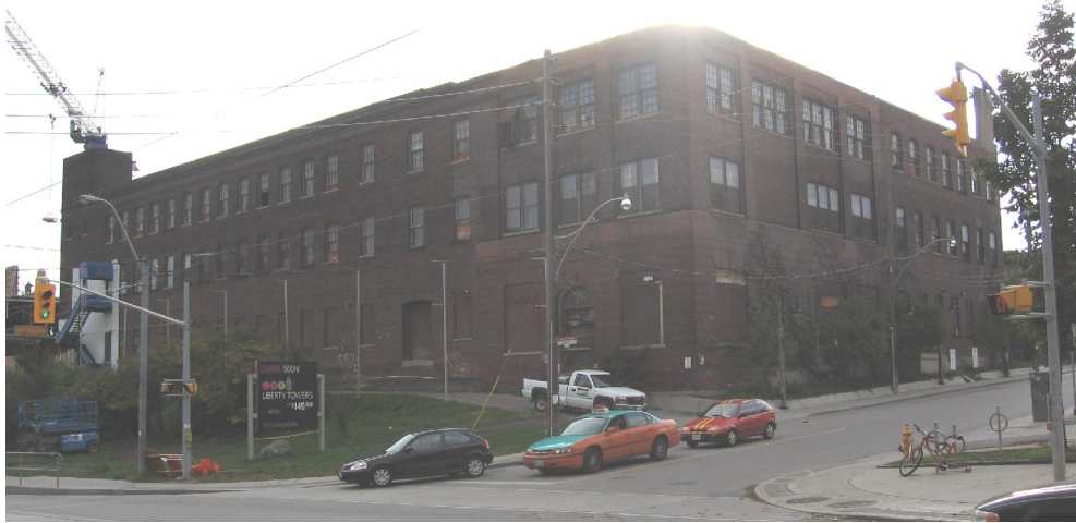
North façade on King Street West (shown on the left)
