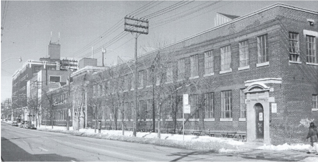
Principal (west) facade
