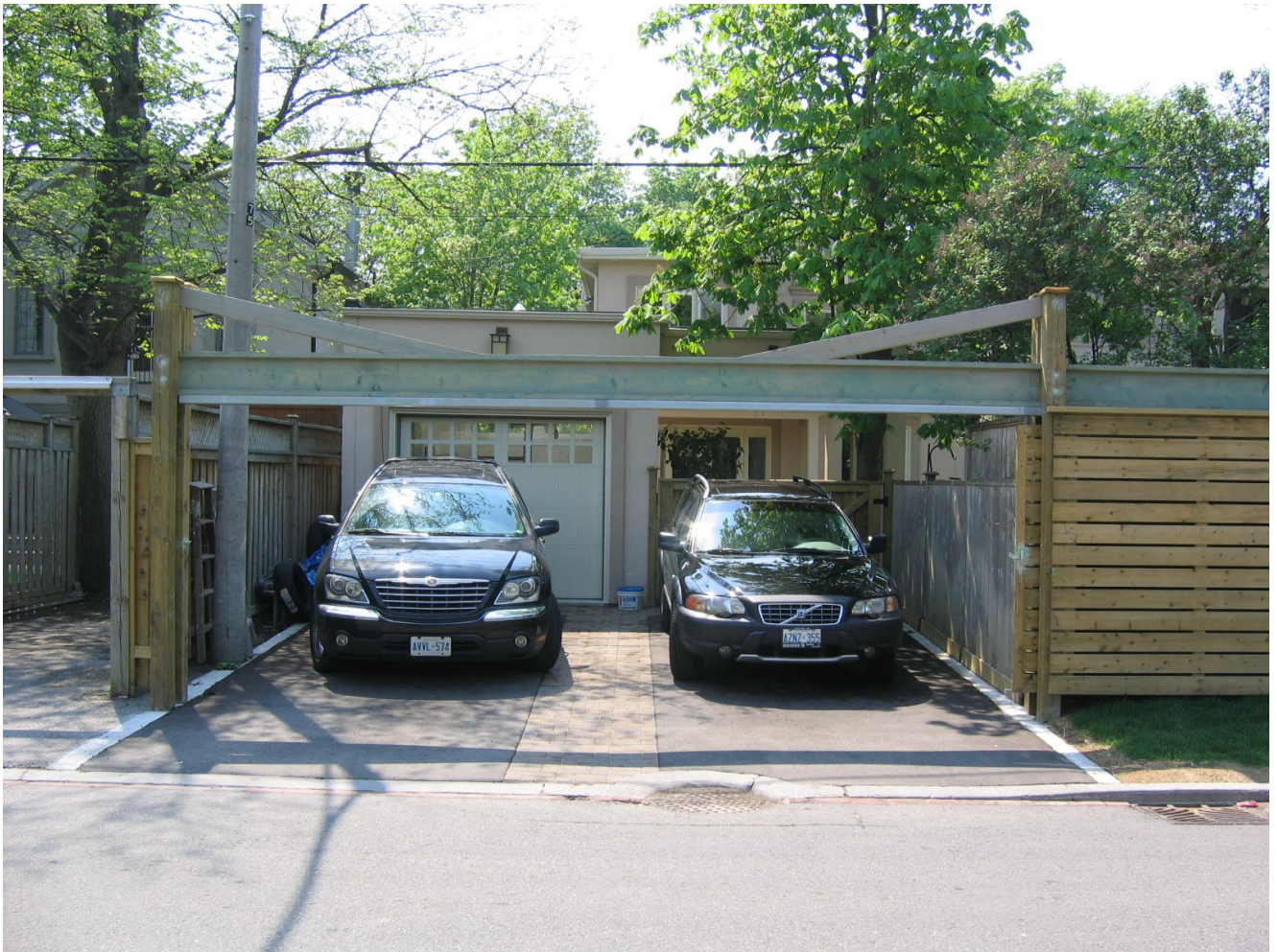
Summerhill Avenue Rear of 26 Whitehall Road
