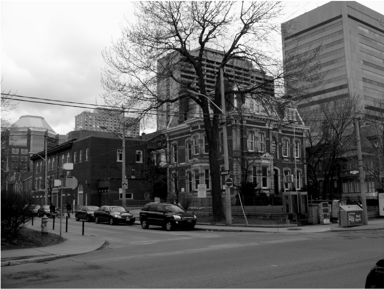
South East Corner View
