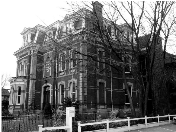
James Cooper House - North East Corner
