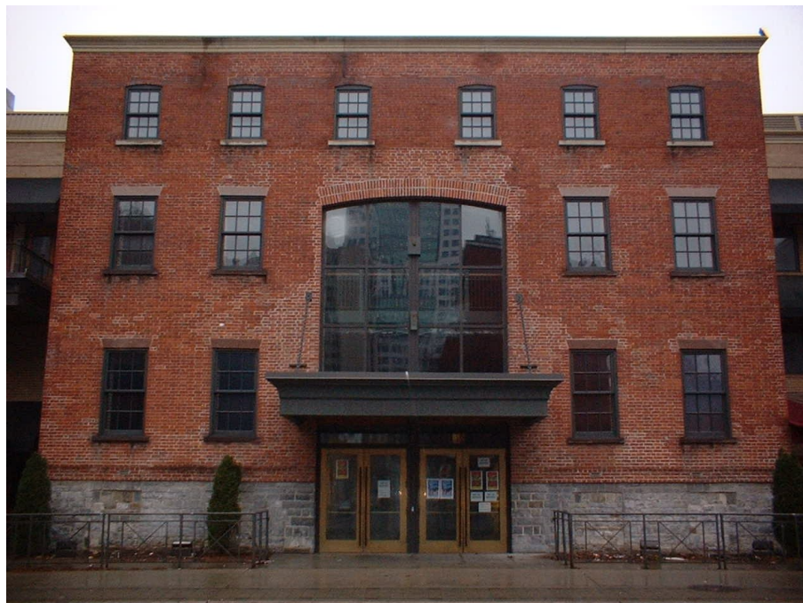
East façade of the George Crookshank House.
