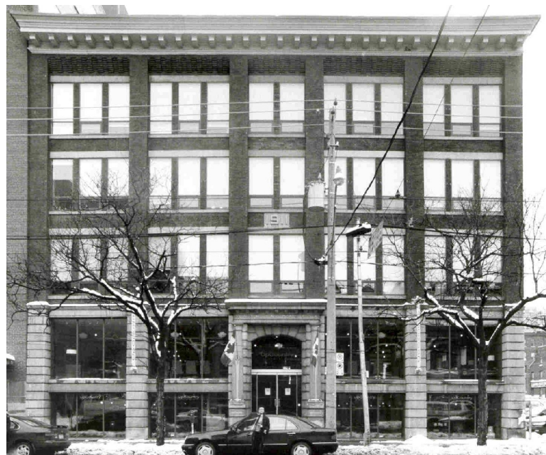
View of the south façade of the W. R. Drummond and Company Dairy Supply Warehouse.
