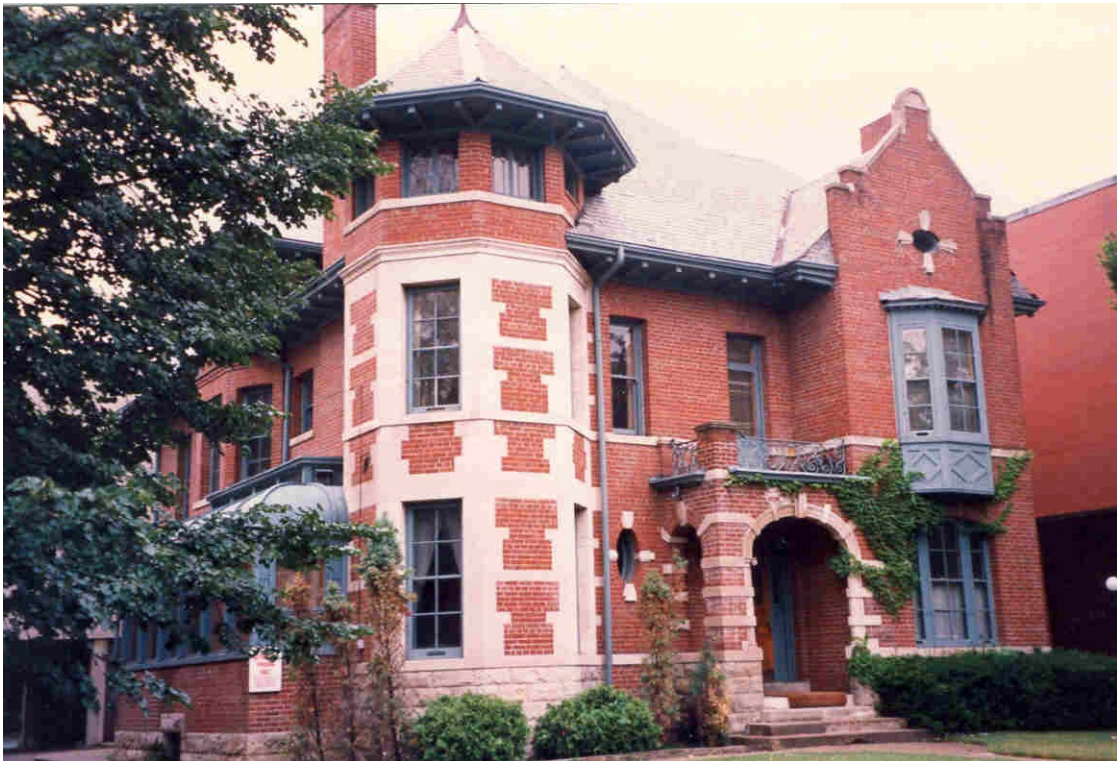
View of the east façade (right) and south elevation (left) of the Robert Watson House.
