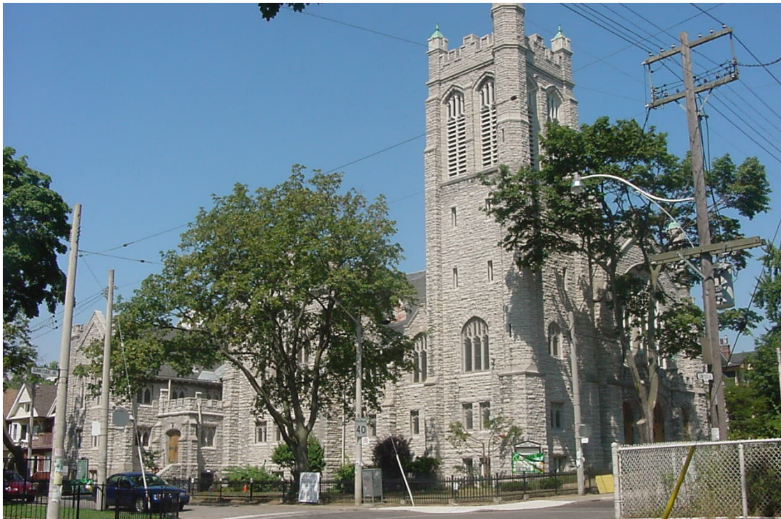
View of Howard Park Methodist Church, showing the east (right) and south (left) elevations, before the building was converted into a residential condominium.
