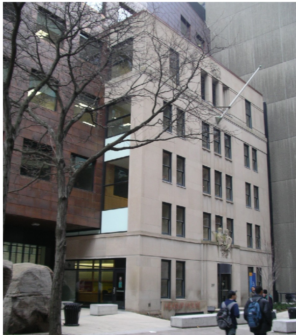
This view of O'Keefe House shows the incorporation of the west façade (right) and north elevation (left) in Heaslop House, Ryerson University.
