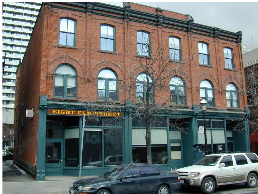
Principal (south) facades of the James Fleming Buildings
