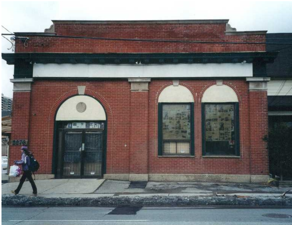
Photograph of the Lake Simcoe Ice Company Office Building, prior to the relocation of the main entrance as part of the redevelopment of the site
