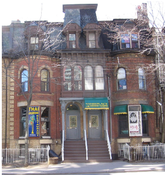
Principal (east) façade of the John Lavelle House (left)
