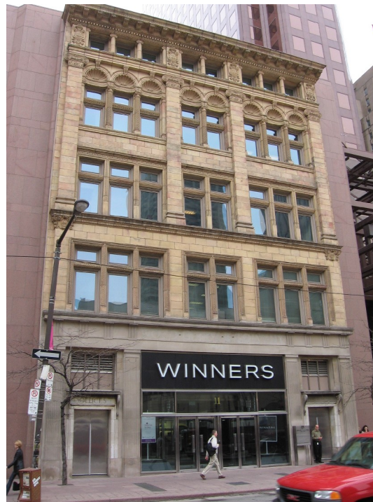
Principal (north) façade of the John McKay Store
