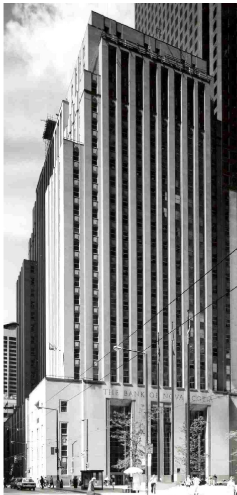
Principal (south) façade of the Bank of Nova Scotia Building
