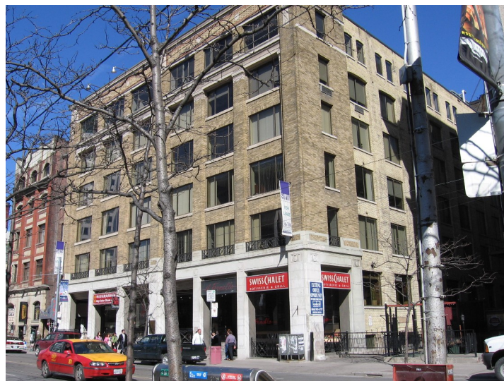
Principal (south) façade of the Canadian General Electric Building
