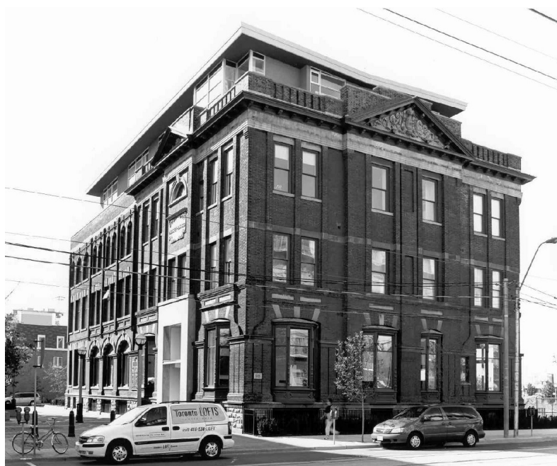
East façade (left) and north elevation (right) of the Massey-Harris Office Building
