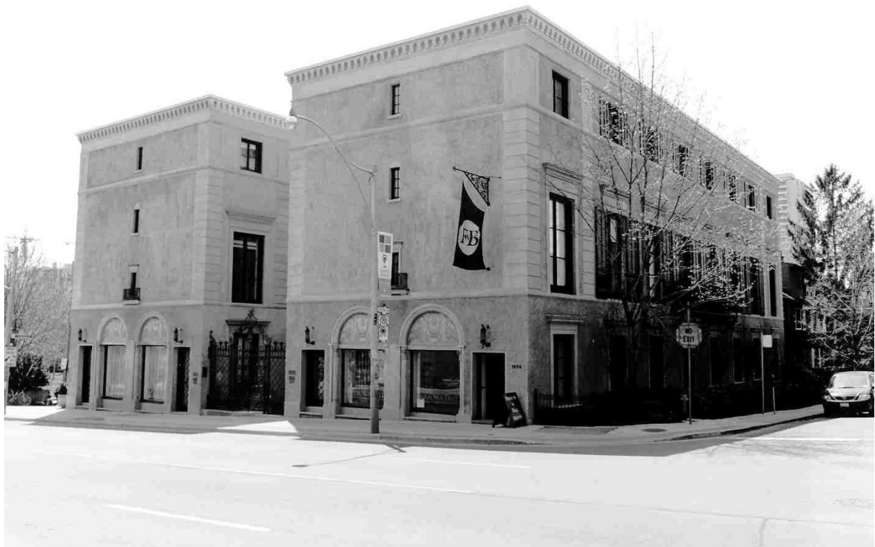
Principal (east) facades of the Crescent Road Apartments
