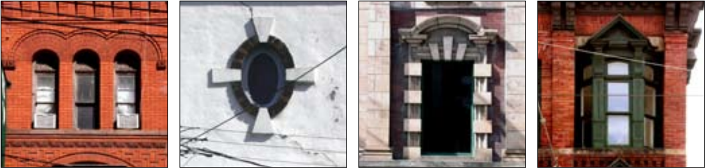
Contributing Buildings on Queen Street West present a wide range of windows, doors and architectural types that contribute to heritage character through their proportion, orientation, and size and scale of elements. Architectural detailing provides a 3-dimensional texture that creates a play of light and shadows on façades.
