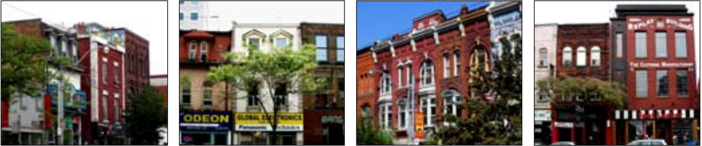
The rooflines of Contributing Buildings create a distinct horizontal edge facing Queen Street West.
