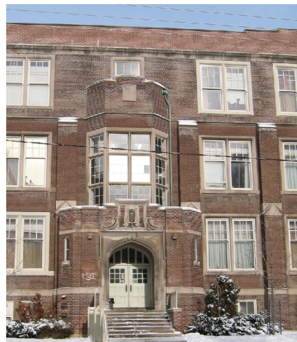
An entrance in the Roehampton Avenue façade showing the third floor addition of 1928 above the original two-storey façade
