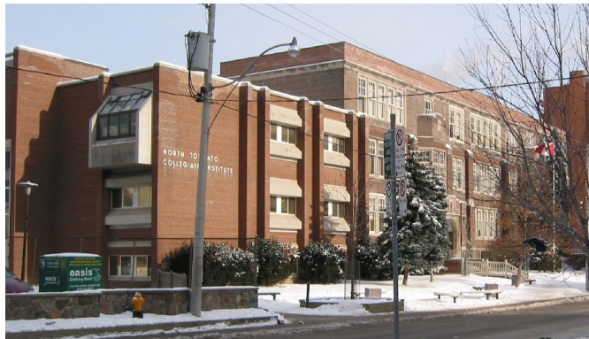
The Roehampton Ave. façade of the 1966 west addition and behind it the original 1921 wing with its 1928 third floor addition
