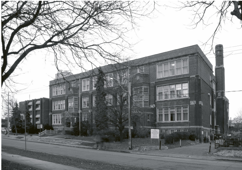
View of south (Roehampton Avenue) façade and east elevation (right) of 1921 wing
