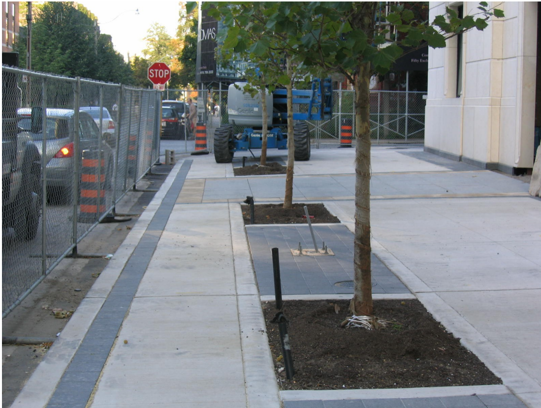
1-11 ST Thomas Street (on Charles Street facing west) September 18, 2007
