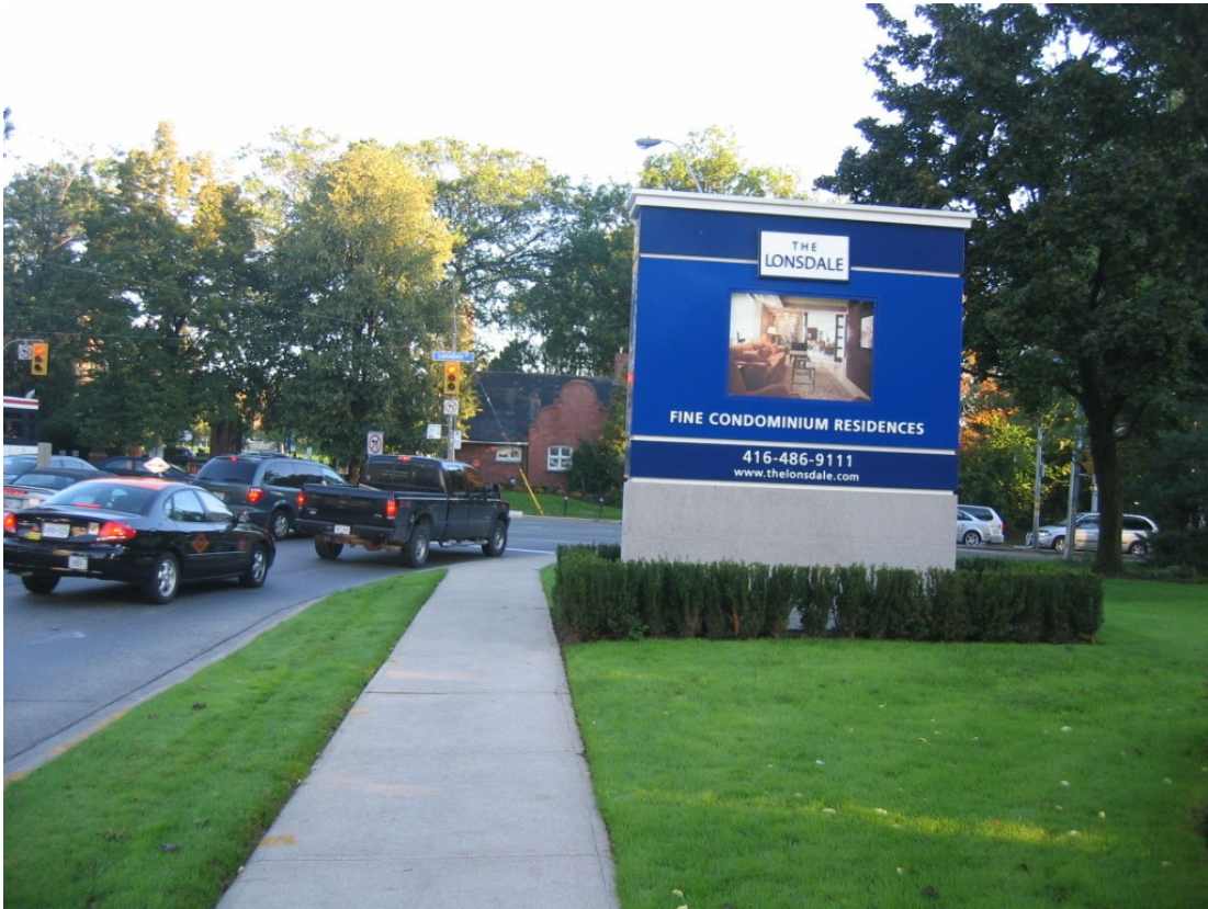
619 & 625 Avenue Road – September 25, 2006
