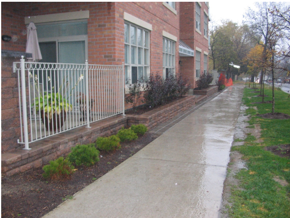
15 Stafford Street - Wellington Street West flank brick retaining wall
