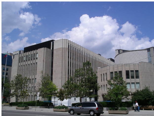
West and South Facades of Courthouse (left) and West Façade of South Wing (right)
