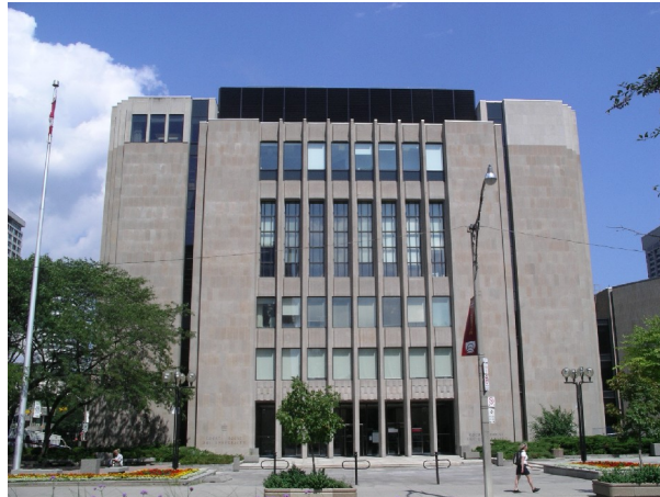
West Façade of Courthouse
