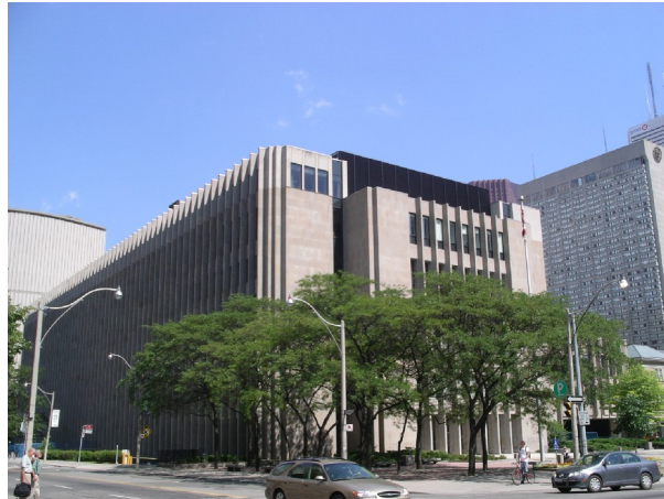
North (left) and West (right) Facades of Courthouse
