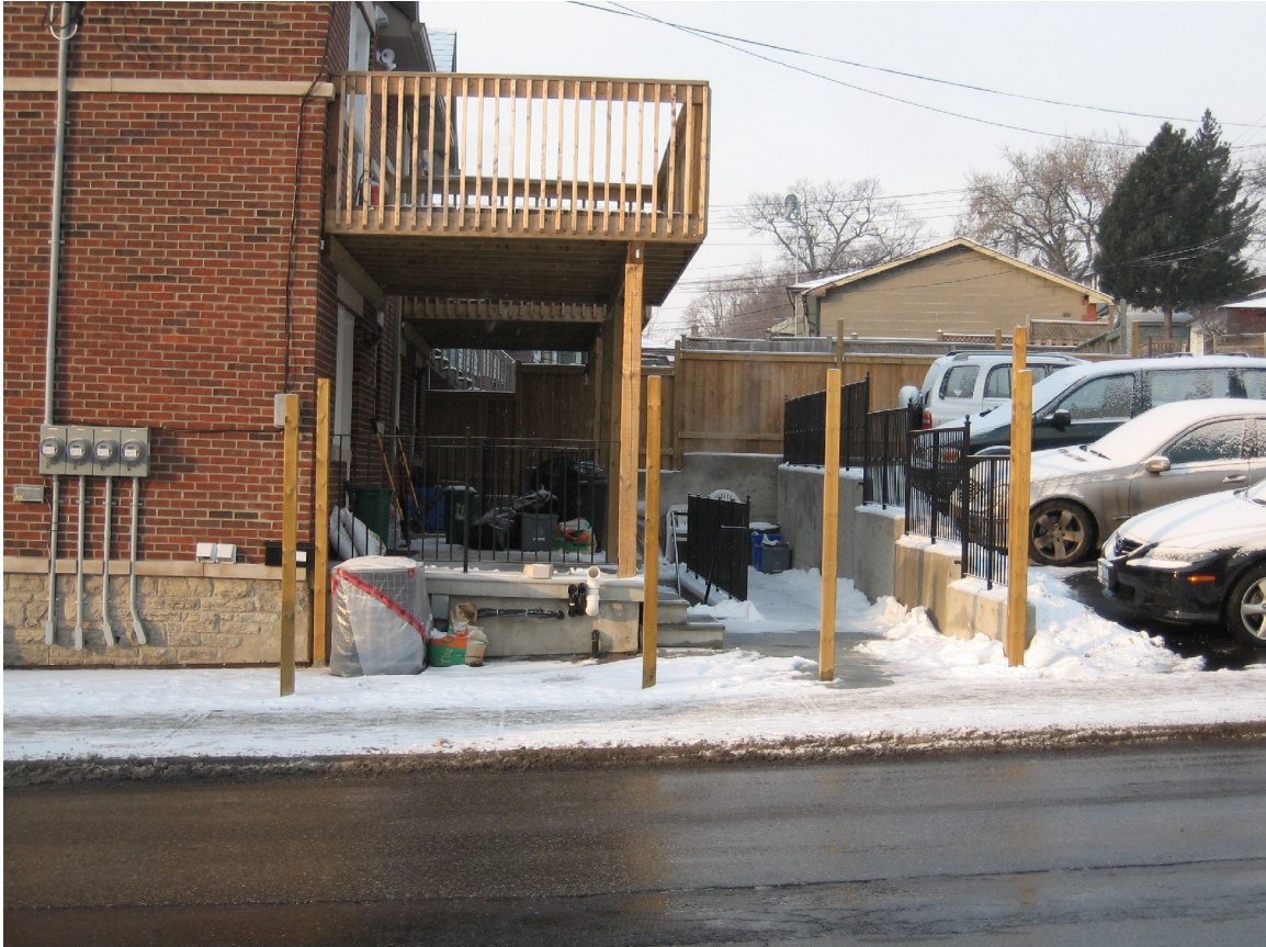
Attachment 8: Photograph looking West on Oakwood Avenue Showing the Proposed Fence Location, the Retaining Wall and the Air-conditioner Encroachments
