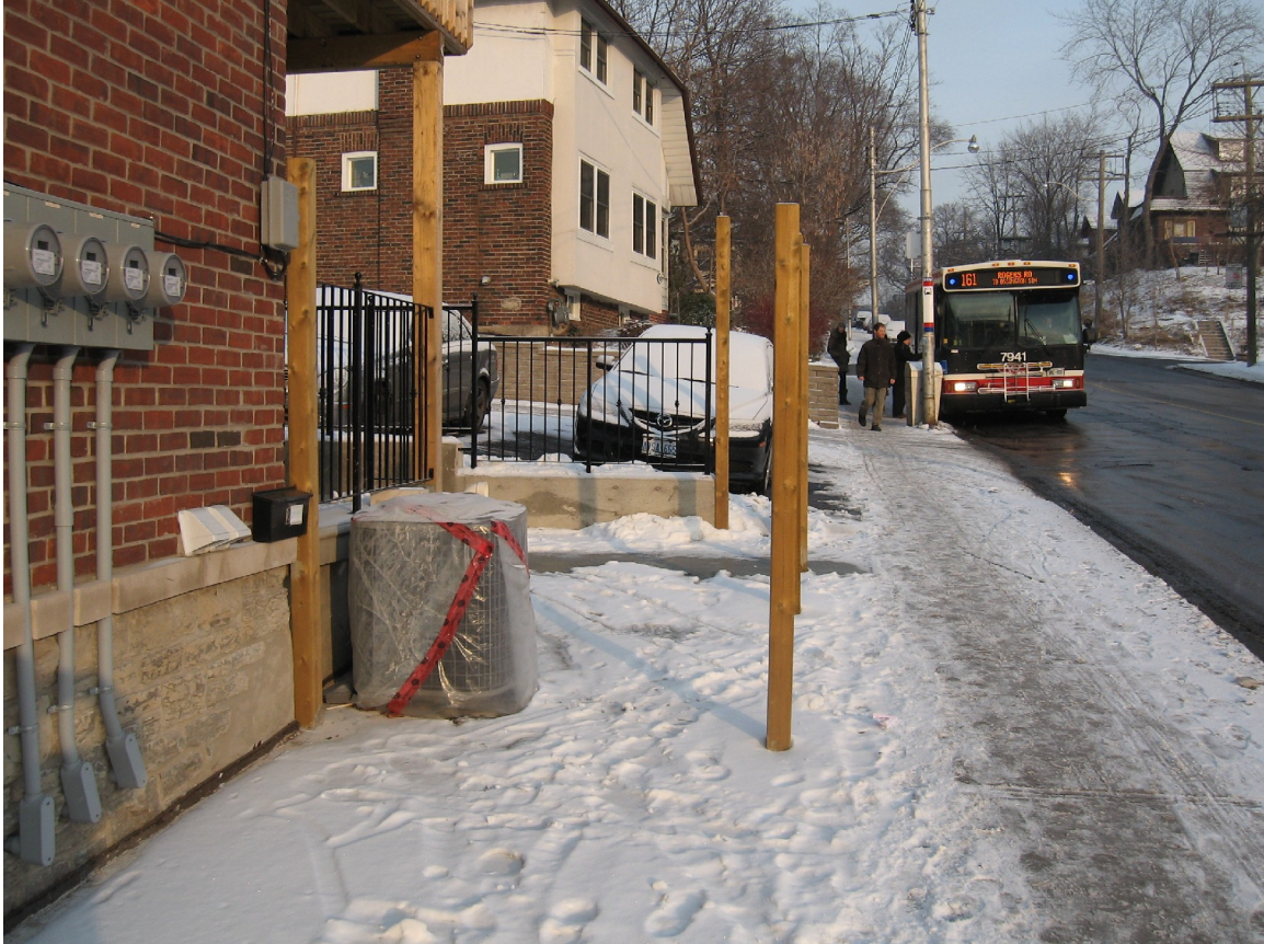
Attachment 7: Photograph looking North on Oakwood Avenue Showing the Proposed Fence Location, the Retaining Wall and the Air-conditioner Encroachments
