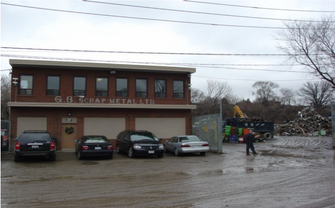
Photograph 1 – Front Elevation of 96 Hyde Avenue
