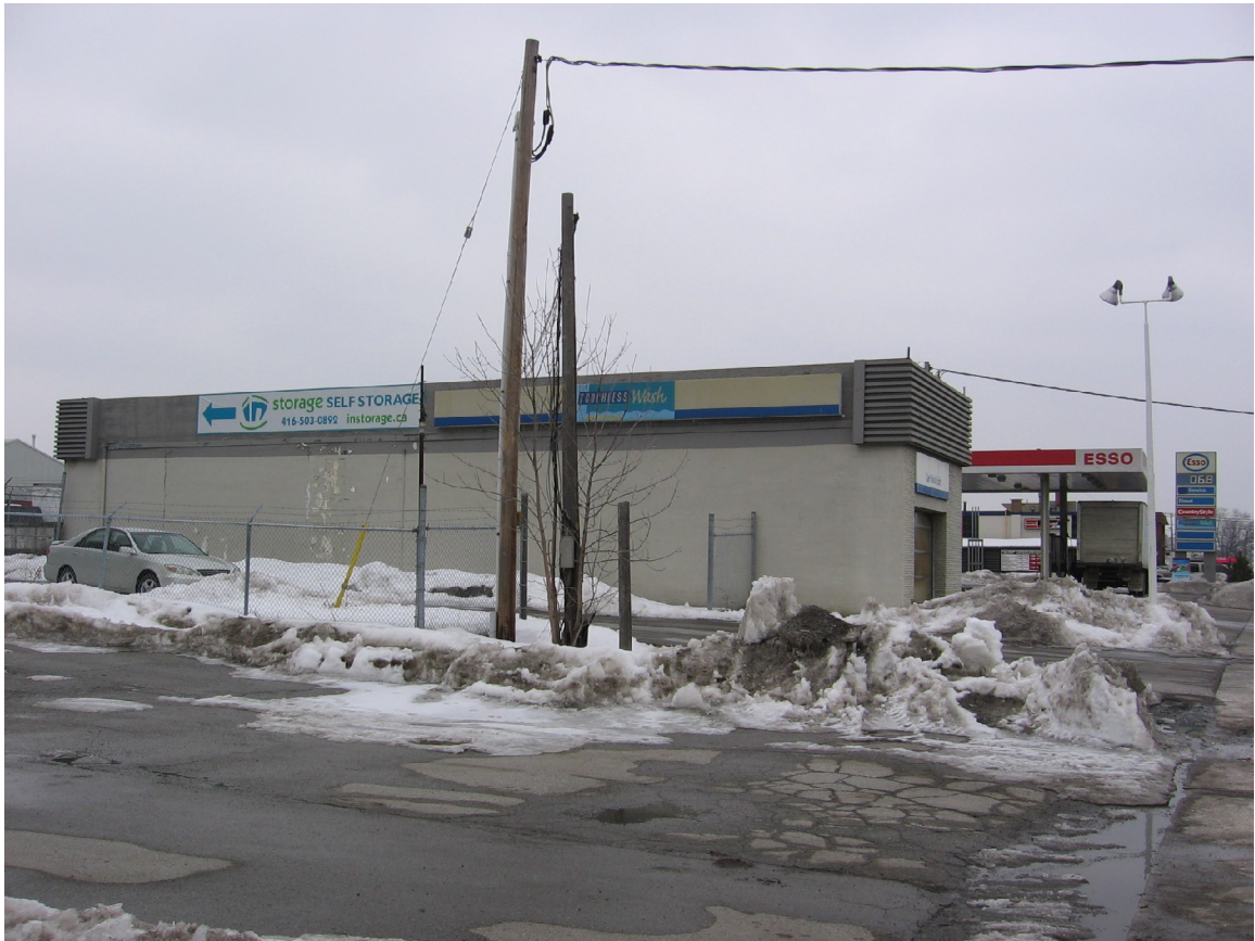
Evans Avenue – North side, East direction
