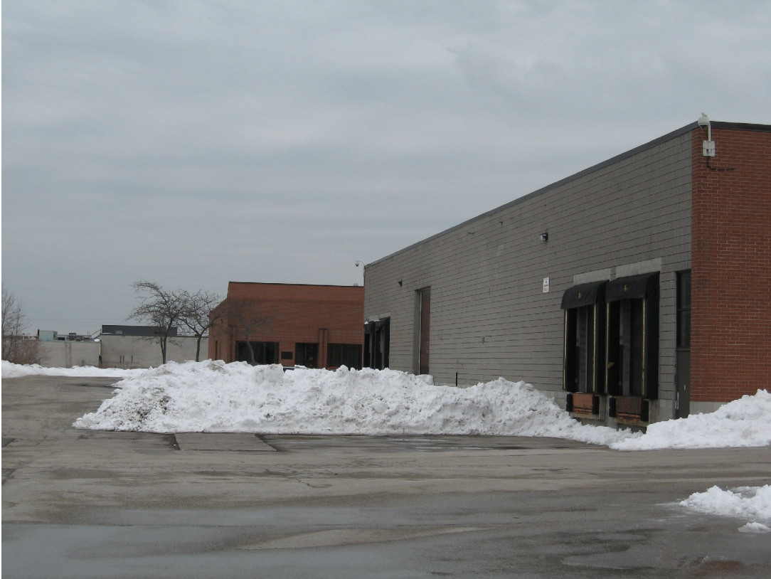
Attachment 6: Photograph of the rear of the building looking south
