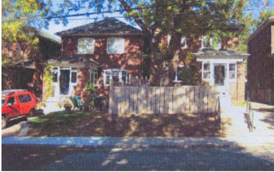
Attachment 3: Photo showing the front elevation of the Fence
