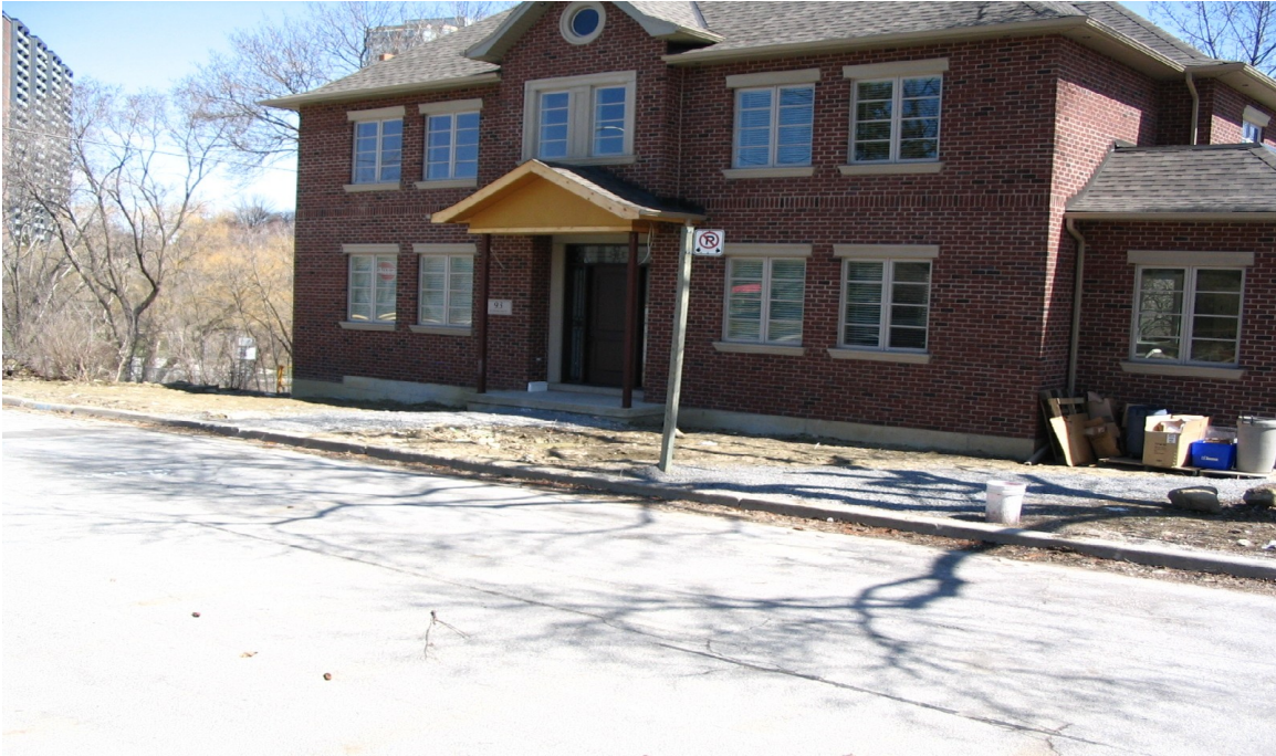
Photo # 1 – Showing the Front Elevation of 93 Raymore Drive
