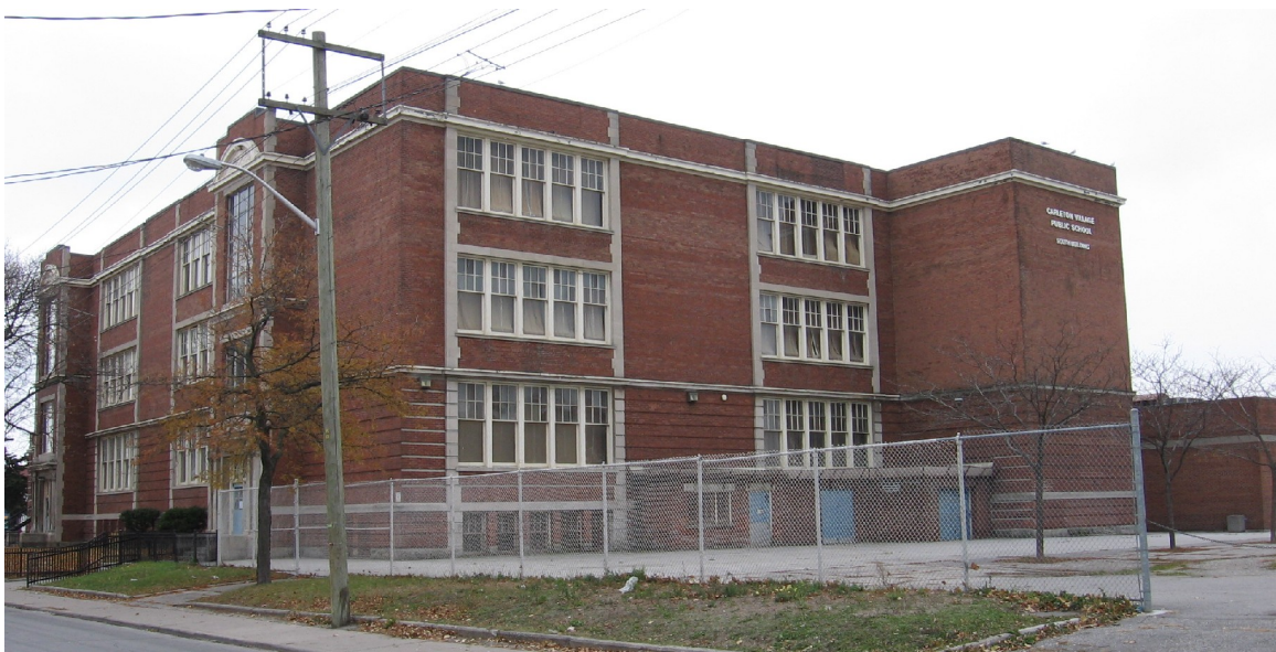
East elevation on left and rear (north) wall on right
