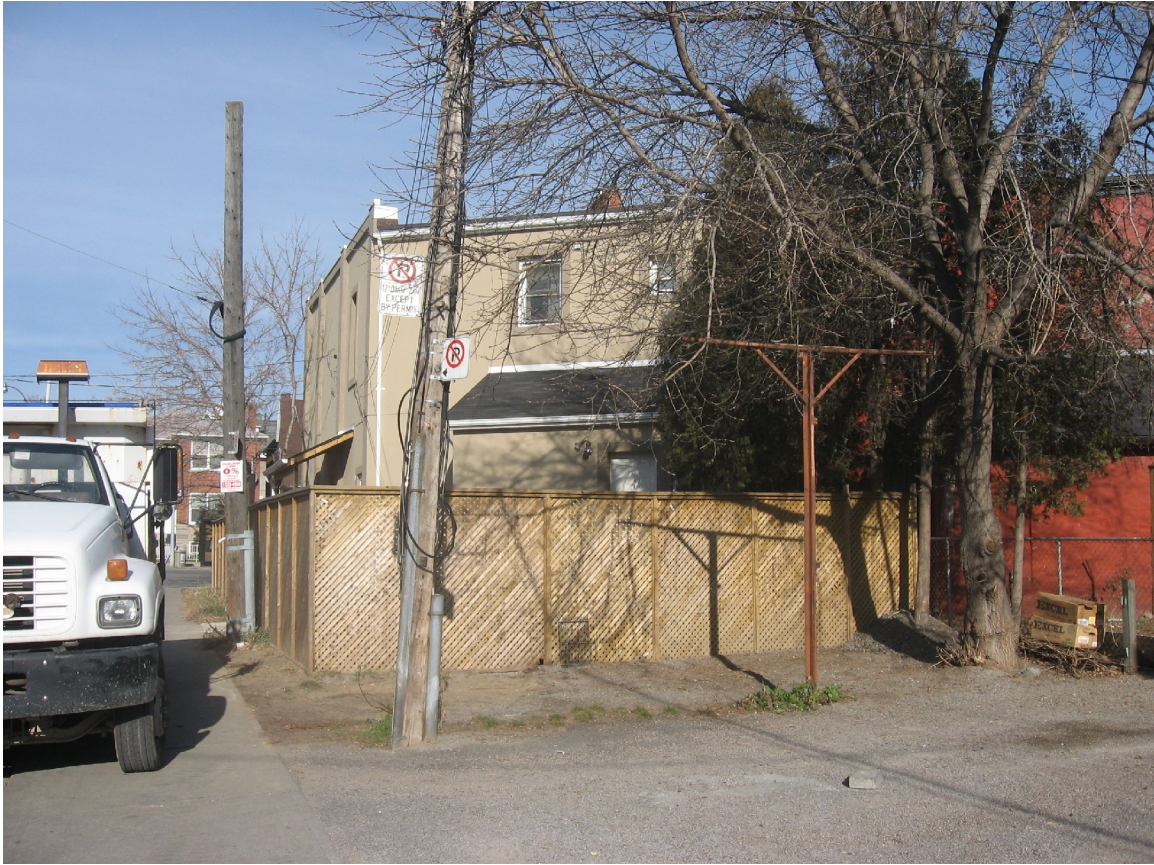
Attachment 4: Photograph showing the south west corner of the encroaching fence which is required to be removed as recommended by Transportation Services
