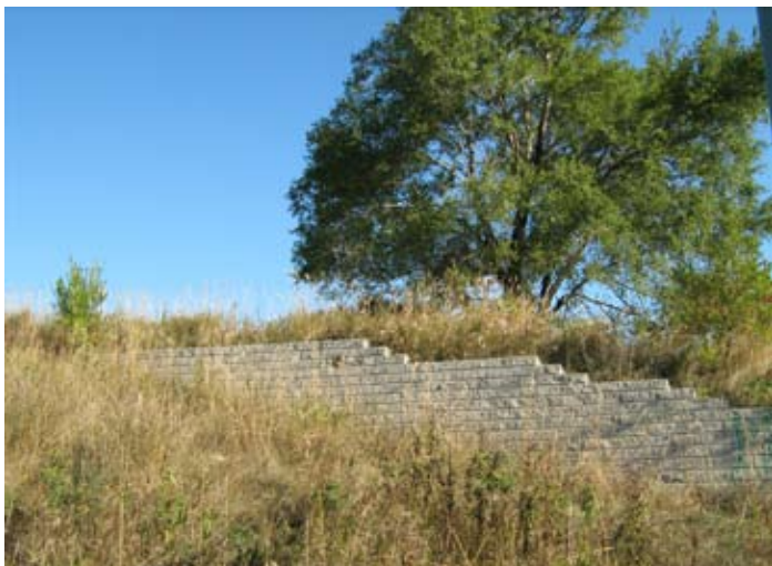
There is a large transition in height that is currently bermed or contained with retaining walls.
