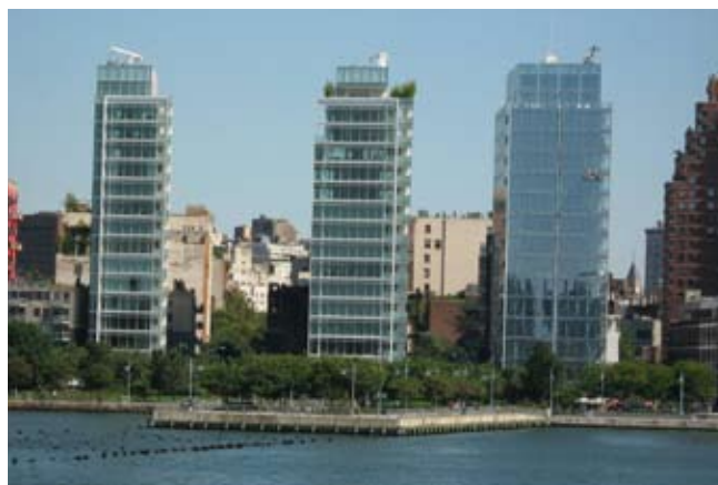
Narrow towers with smaller floor plates maximize views to the lake.
