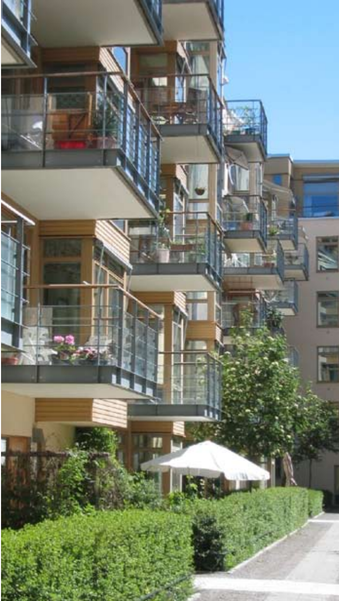
Access to the outdoors and daylight allows buildings to be naturally ventilated and creates positive residential environments.
