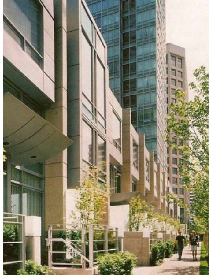
Podium buildings humanize the scale of highrises, resulting in more comfortable pedestrian oriented streets and public space.
