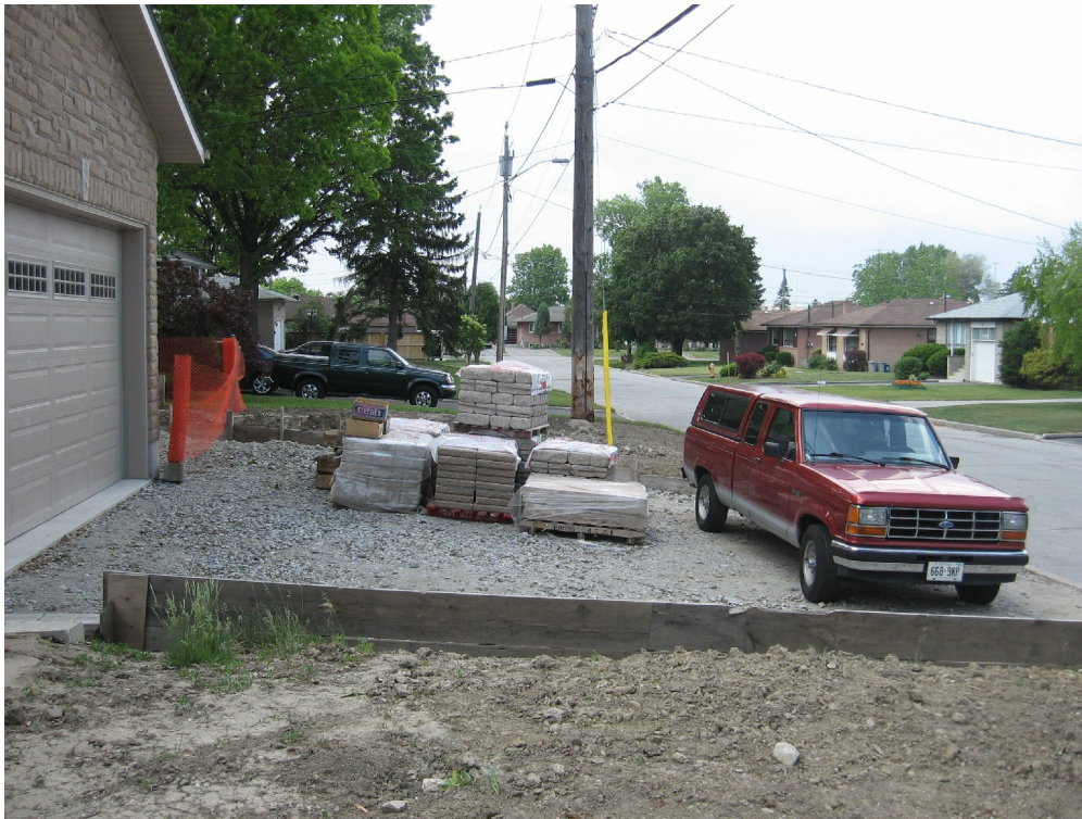
Attachment 2: Photos showing the Portage Avenue flankage
