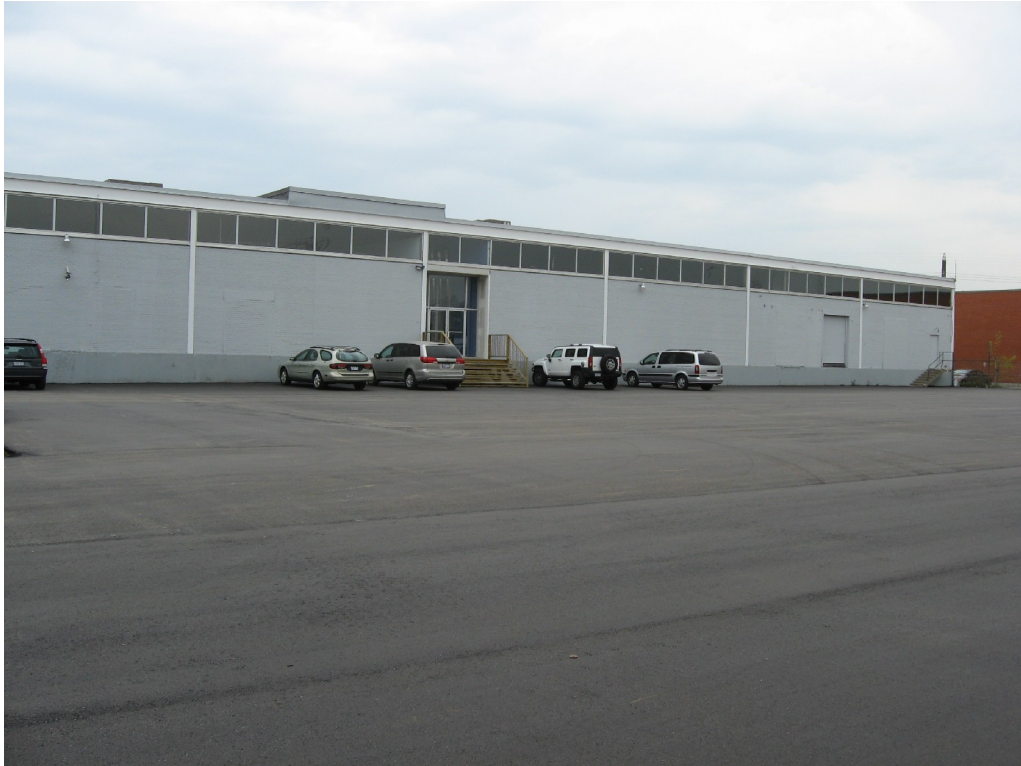
EXISTING REAR WALL AND ENTRANCE
