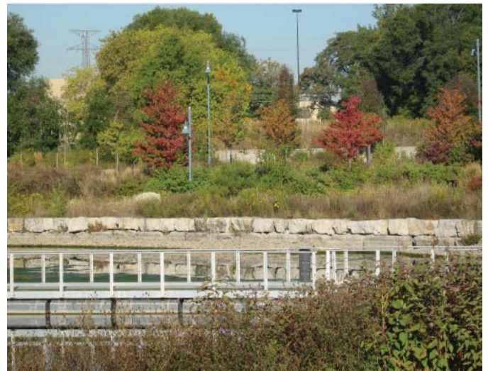
The area benefits from extensive and well established landscaping along the waterfront.
