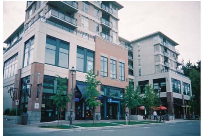
Spaces in podium buildings could be used for community facilities such as daycares, libraries and medical clinics.
