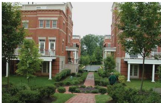
Internal courtyards create safe and comfortable landscaped spaces between buildings.
