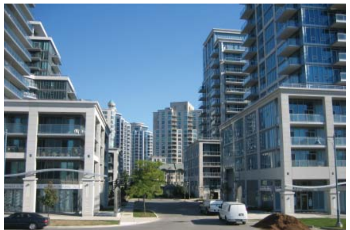
Large floor plates minimize views through the site.
