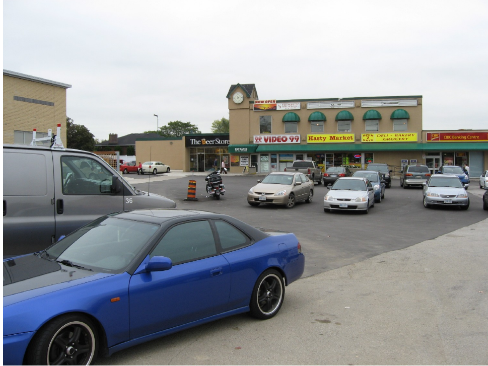
Portion of existing strip mall in the south-east quadrant of strip mall
