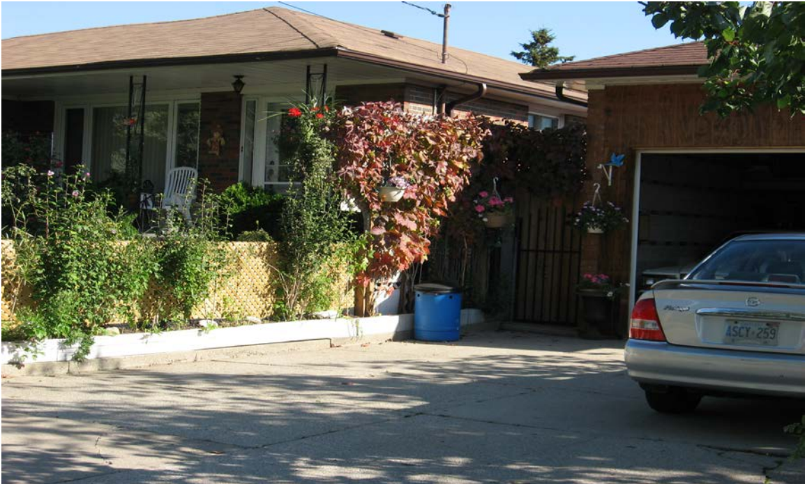
Photo # 2 – Subject Fence/Gate/Lattice Between 33 and 31 Apted Avenue
