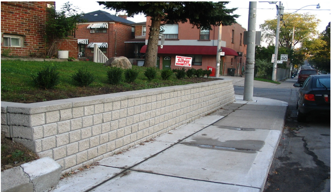
Photograph # 2 - Retaining wall encroachment on Hope Avenue road allowance
