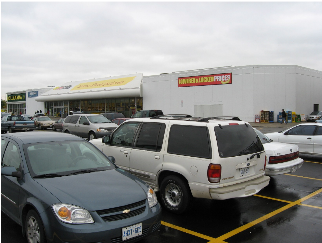
Building just to the east of the plaza where Shoppers Drug Mart is located in
