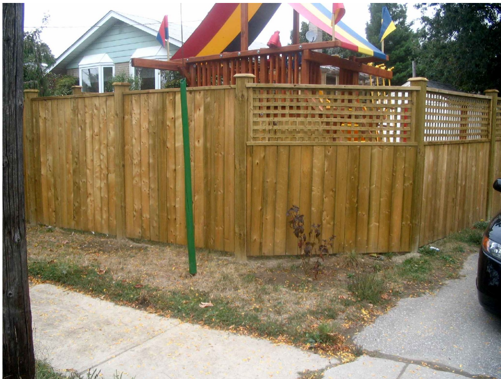
Attachment 6: Photos showing the fence with traffic sight line problem
