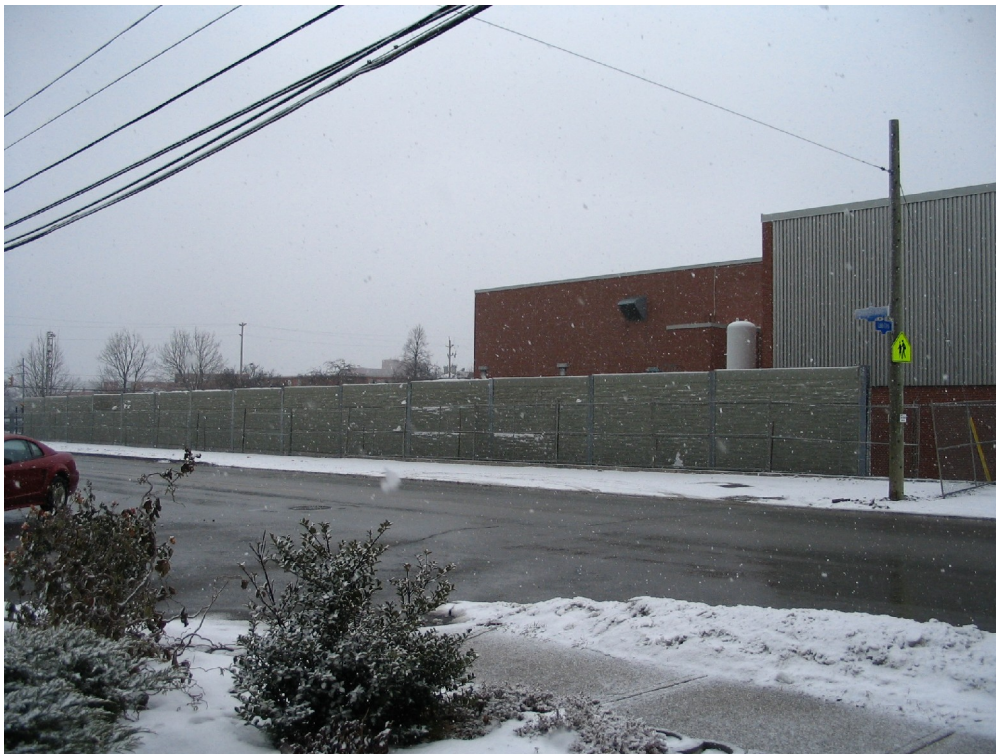
Attachment 5: View of Loading/Unloading Area before (above) and after (below) installation of Noise Barrier Wall on Dwight Avenue
