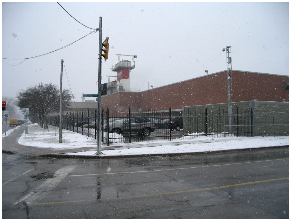
Attachment 6: Photos showing the Wrought Iron Open Grille fence at Dwight Avenue and Birmingham Street
