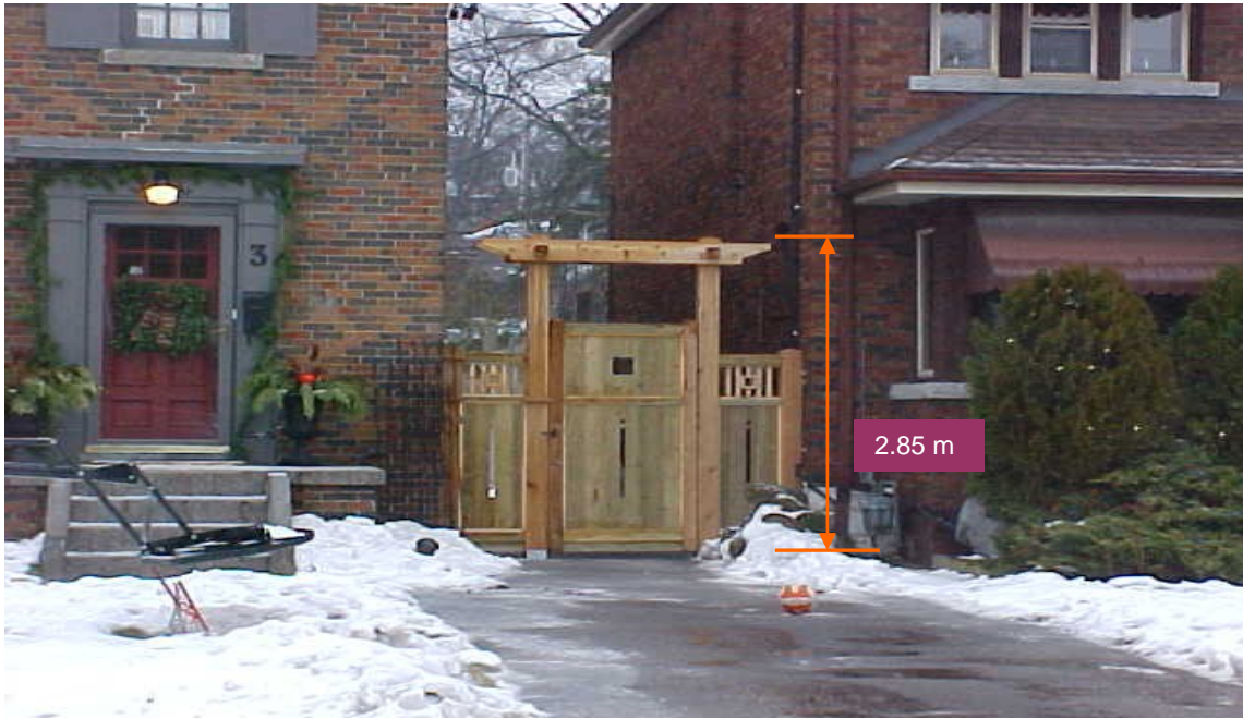
Photo of Gate Structure
