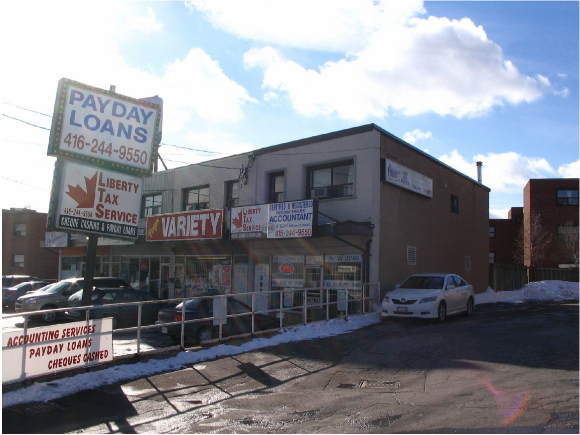
2266 Keele St - North end of a strip of 4 buildings
