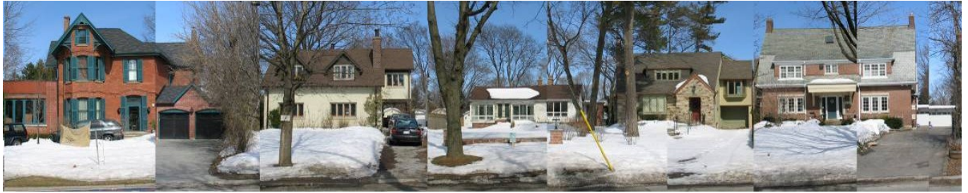
Existing streetscape with 112 in the centre.
