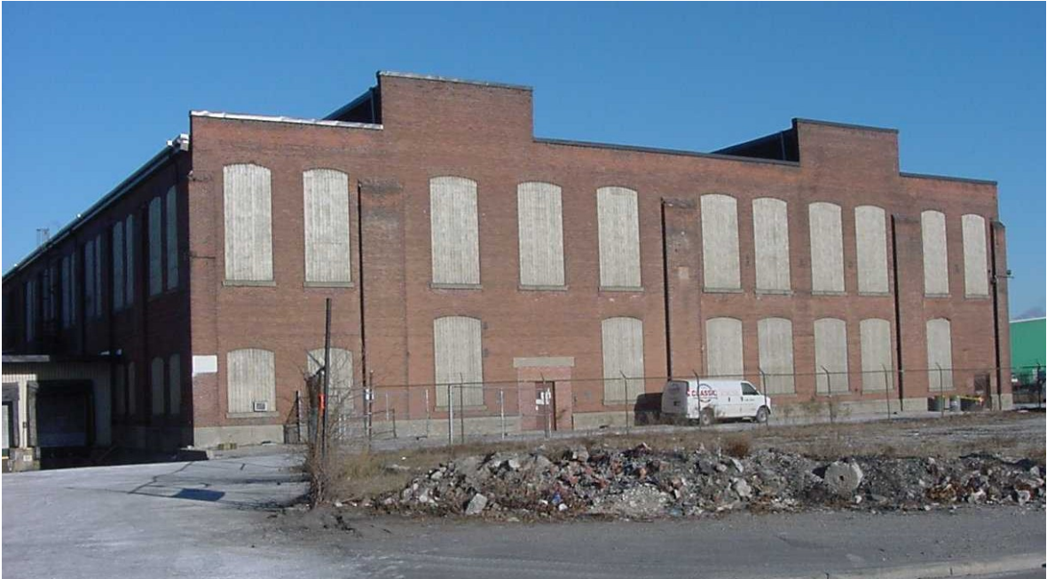
View of the south façade facing Esandar Drive
