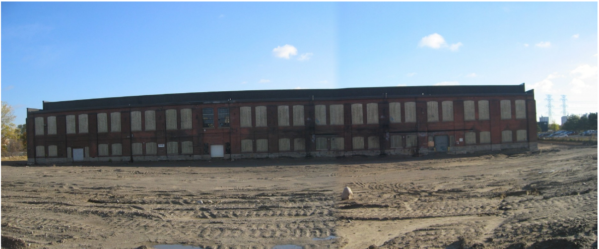
View of west façade facing Laird Drive
