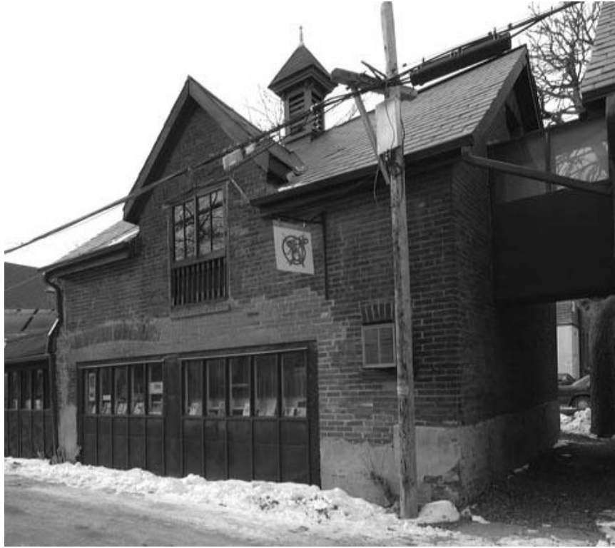
South Coach House, showing the east elevation on bpNichol Lane
